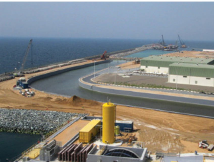
Hamriya Power Station, Sharjah, UAE
